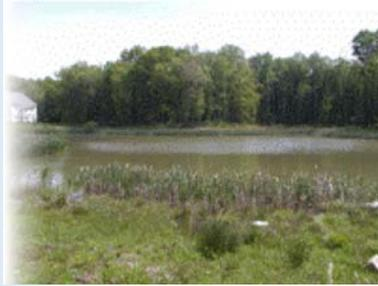
Wet ponds have a fairly standardized design that is specially aimed at managing and treating stormwater. These ponds stay wet year round. Stormwater only discharges from the pond when the water level rises over the outlet after pollutants settle in the pond.
