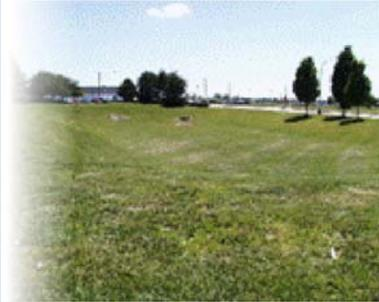
Dry ponds are stormwater runoff containment areas that remain dry except after rain. After the runoff is conveyed to them, an outlet structure allows stormwater runoff from a recent storm to slowly drain into a nearby waterway.
