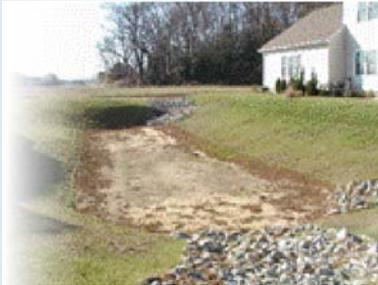
Infiltration basins collect stormwater runoff in the same manner as wet and dry ponds, but they do not release the water through an outlet structure. Infiltration basins are designed so that stormwater eventually soaks into the ground, trapping pollutants, imitating natural conditions, and recharging groundwater supplies.
