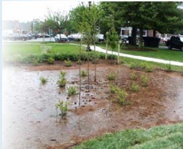
Scientists and engineers are currently designing and promoting new stormwater management devices that mimic nature and require much less maintenance. One example is the bioretention cell. Although it has the appearance of a landscape island, it is designed to temporarily store and treat stormwater runoff.
